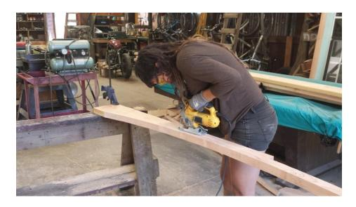
After gutting the car, the crew went to work replacing the roof. We tore down the old sheathing, revealing a rotted skeleton. We then created a template with one of the intact rafters using discounted materials from Fort Jones Lumber, a local company, and re-created the rafters which would ultimately hold up the new roof.
