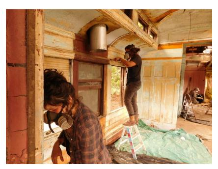
Lead abatement during the deconstruction of the car was also of great concern, so during this process we worked to ensure that our volunteers were safe and that all the paint chips were properly disposed of. The windows were also removed in order to scrape off the lead paint and determine which frames could be salvaged and which would have to be replaced. Luckily many of the etched top-windows remained intact, which we can then use to recreate the ones that did not survive.
